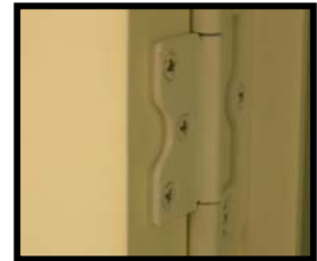
Hinge spacer installed.
