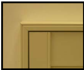
Ensuring the reveal is even.
