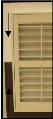
Loosen screws on panel hinge. Do not remove completely.
