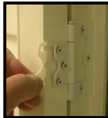
Insert hinge spacer.
