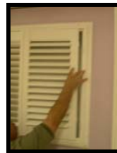
Insert panel into position.
