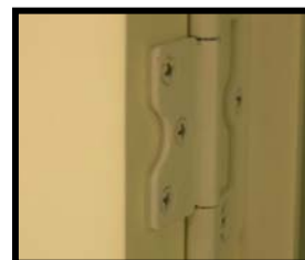
Hinge spacer installed.
