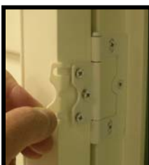
Insert hinge spacer.
