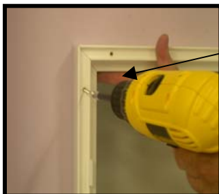
Only secure one screw into the top left frame.
