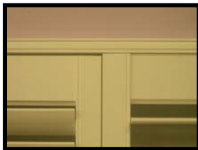
Once you have installed the panels, and they do not line up,
