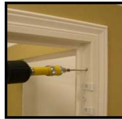
Only secure one screw into the top right frame.
