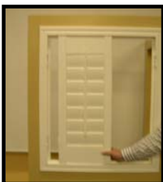
Position panel in the frame.
