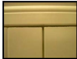
After racking of shutter, panels should line up.
