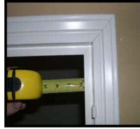
Measure Left & Top frame for spacing.
