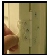
Insert spacer behind hinge.
