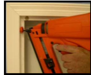
Only secure one screw into the top left frame.
