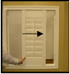
Position panel in the frame.
