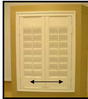
RACK the bottom of your frame to the left or right for an even reveal.
