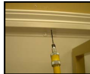
Pre-Drill middle of top and bottom frame.
