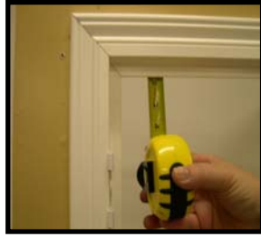
Measure Right & Top frame for spacing.
