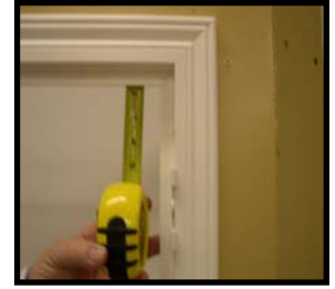
Measure Left & Top frame for spacing.
