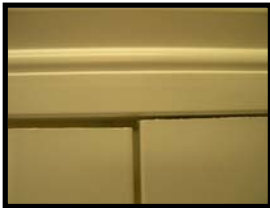
Once you have installed the panels, and they do not line up,
