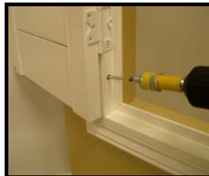
Pre-Drill bottom right & left frame.
