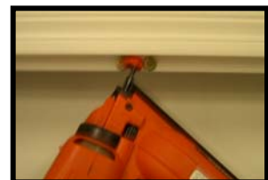
Only secure one screw into the top frame.
