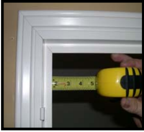
Measure Right & Top frame for spacing.
