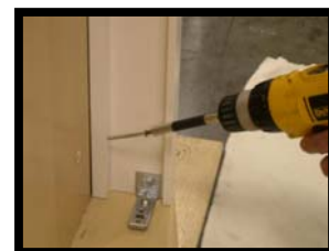
With PIVOT Leg Straight and LEVEL, screw Leg to the Wall
