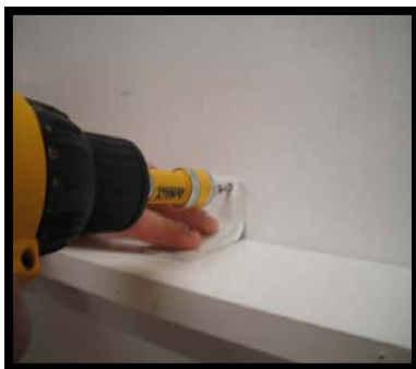
Install Bracket onto Header (Flush with the wall)
