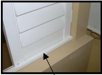
First, install bottom light block.
