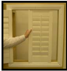
Panel in the window opening.
