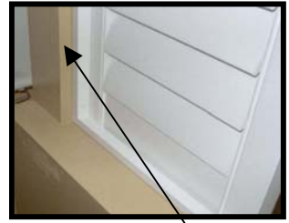
Finish by installing left light block.
