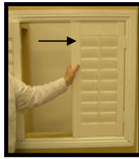
Slide panel to left window jam.
