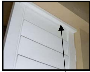
Follow by installing top light block.
