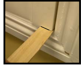
Push shim until stile is in line with shim mark.
