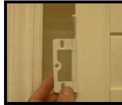
Completely install the hinge pin.
