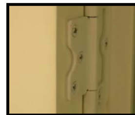
Hinge spacer installed
