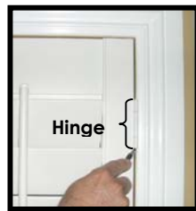
Mark should be made on the wall/jamb at the bottom of the hinge.
